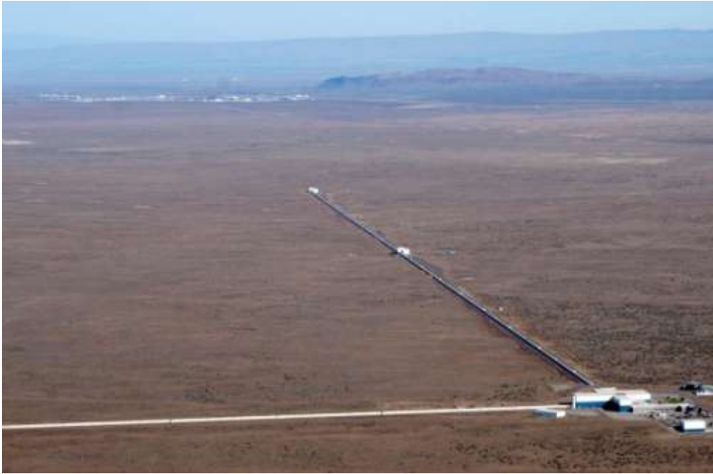
One of the two American LIGO facilities 20 .
