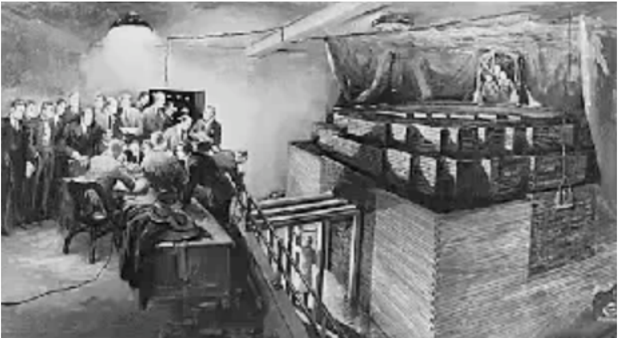
Control of the reactor with cadmium bars.
